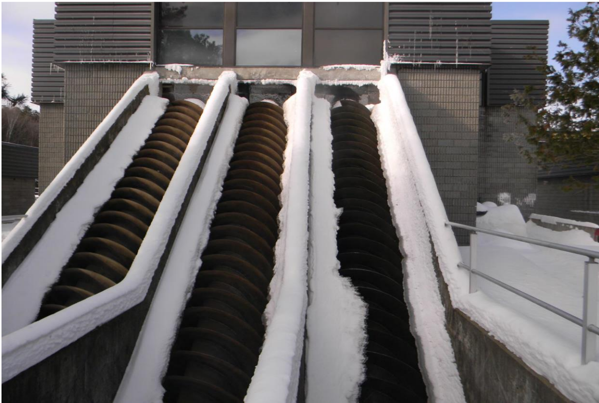
Figure 3 - Wastewater Treatment Plant (Screw Pumps)
