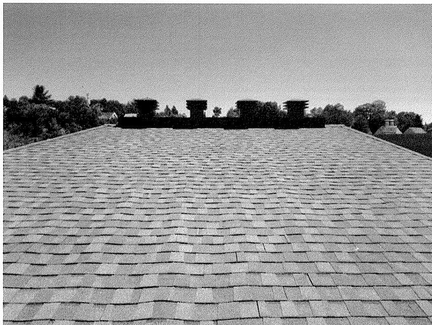
Figure 4: Roof field above pool and men's changerooms (Phase 1 replacement).
