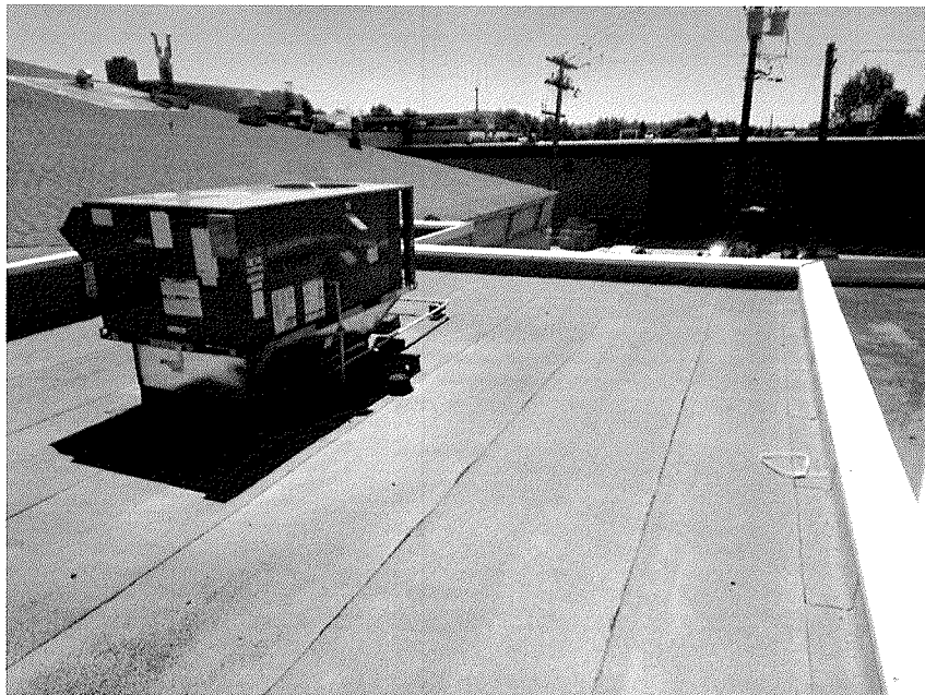
Figure 2: Existing torched-on roof membrane, Exercise Room (Phase 2 replacement).
