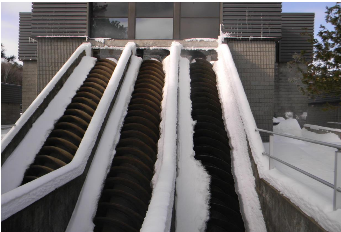
Figure 3 - Wastewater Treatment Plant (Screw Pumps)
