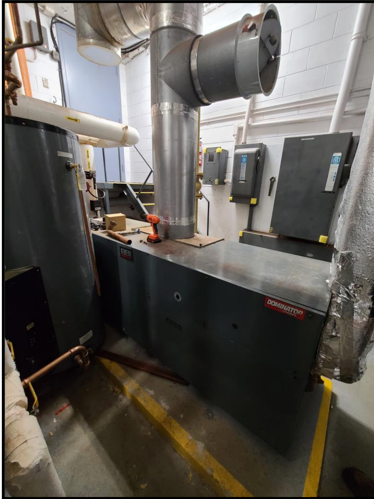
Fig. 2.3.1: RBI Hot Water Boiler
