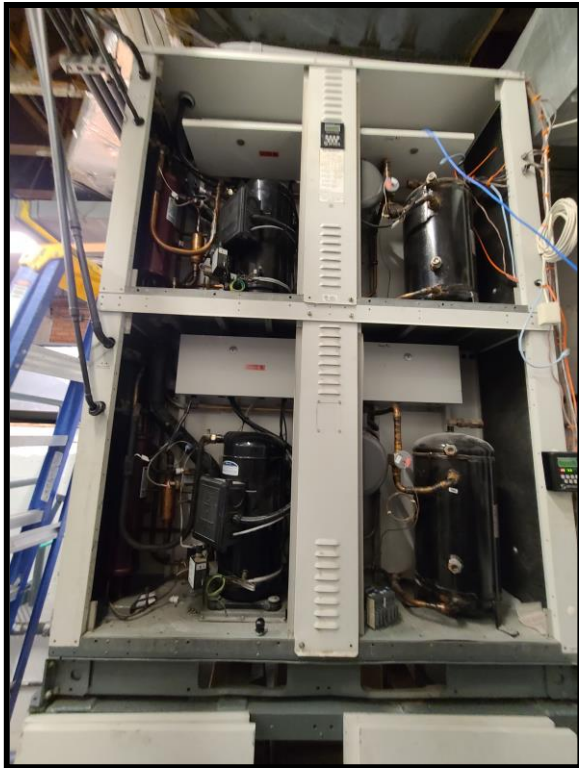
Fig. 2.2.1: Compressors inside Seresco Unit
