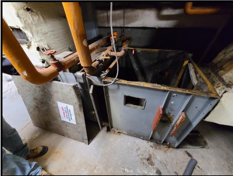
Figure 2.4.1 Redundant Air Handler
