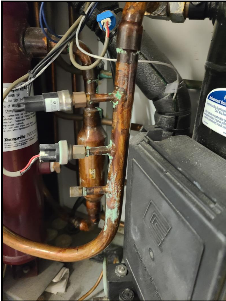
Fig. 2.2.4: More corroded piping inside unit
