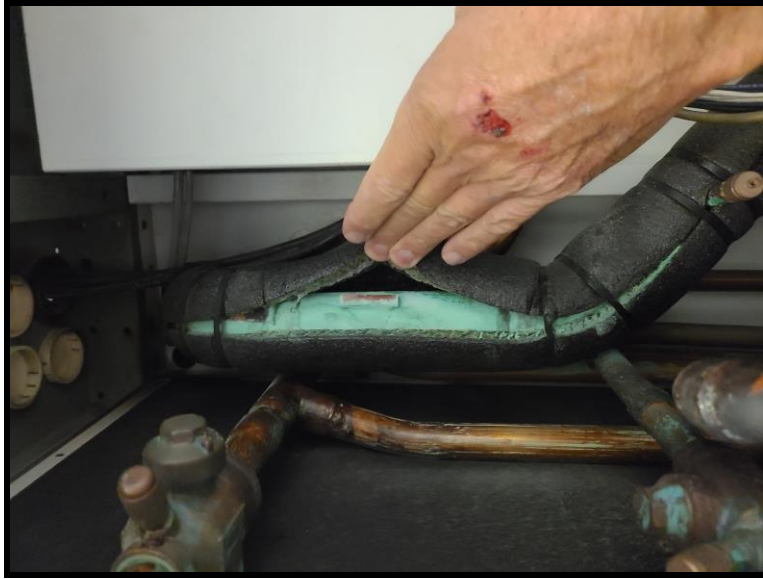
Fig. 2.2.3: Example of Corroded piping in Seresco Unit
