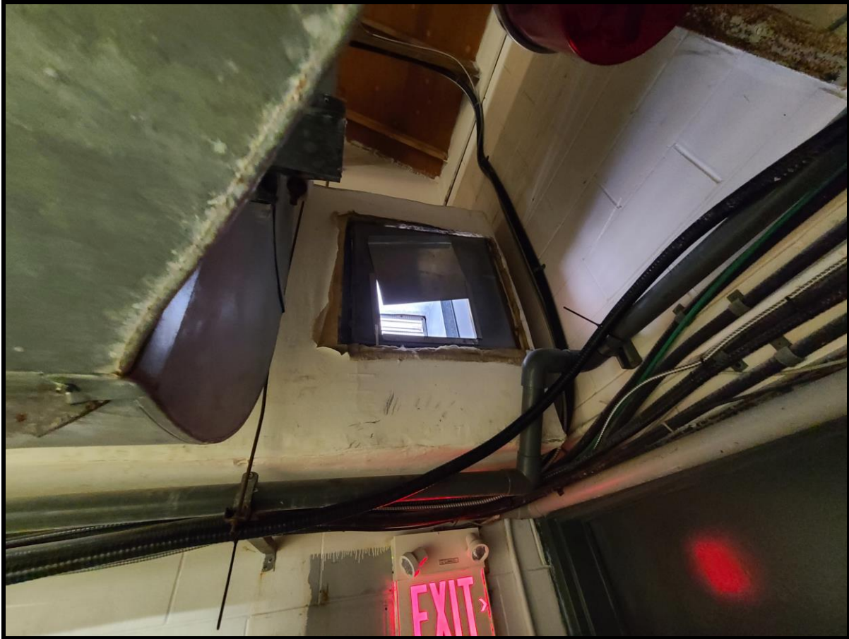
Fig. 2.2.5: Temporary opening in ductwork
